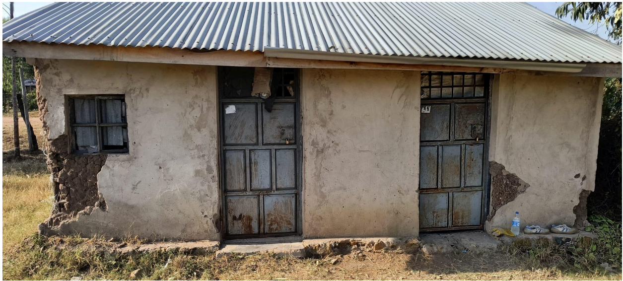
Photo 3: Hut of the worker and storage for seeds.
